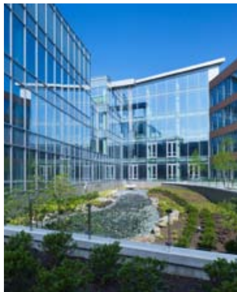
Buildings surfaces can be the first step in the overall slowing, sinking, and storing regime
